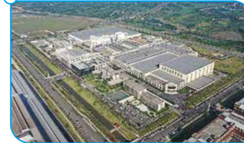
On May 28, 2022, the production line of 150,000 tons of glass fiber chopped strands produced by Jushi Chengdu Intelligent Manufacturing Base was successfully started up, and the entire Chengdu Intelligent Manufacturing Base was completed.
