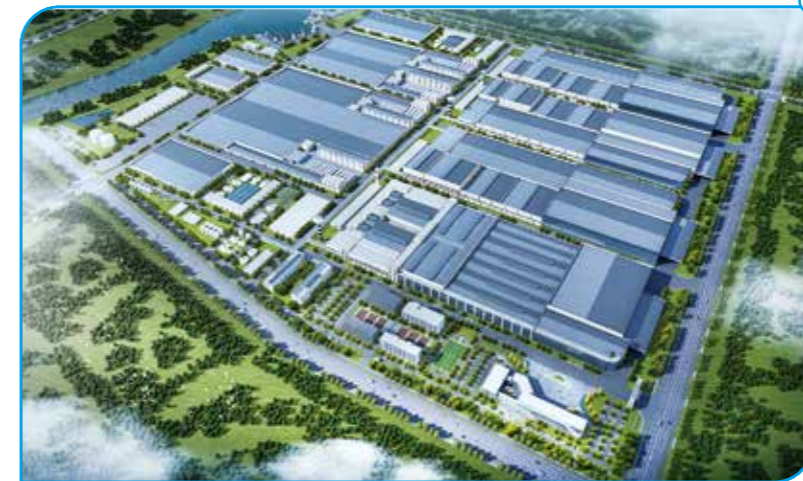
On February 8, 2023, the foundation of China's Jushi Huai'an Lianshui Glass Fiber Zero Carbon Intelligent Manufacturing Base was laid and the first phase of the project officially commenced.
