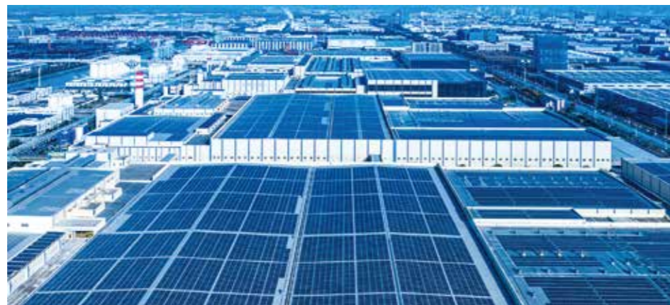
A 600,000 square meter roof in Tongxiang, achieving full coverage of solar photovoltaic panels for the company, generating nearly 70 million kWh of electricity annually, all used for production.
